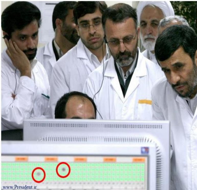
Figure 3: Former president Ahmadinejad looking at SCADA screens in the control room at Natanz in 2008. The screen facing the photographer shows that two centrifuges are isolated, indicating a defect, but that doesn't prevent the respective cascade from continuing operation (highlighting in red not in the original)
